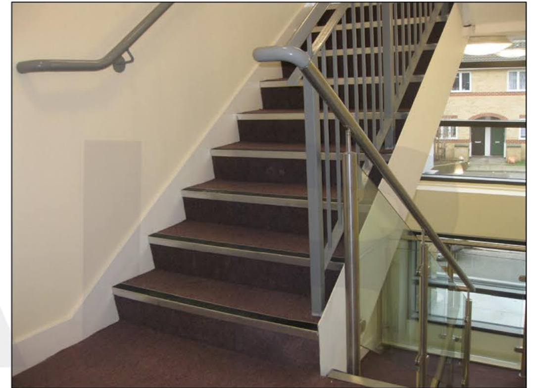
Picture shows finished stair on site with site welding completed at landings, and paint applied.
